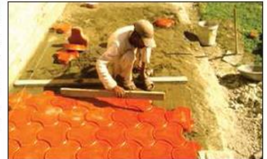
Manual laying of Paver blocks in Institute Premises (M30)
