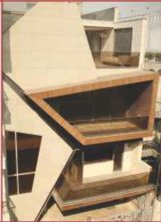
Exterior Facings- The Taper House, Delhi
